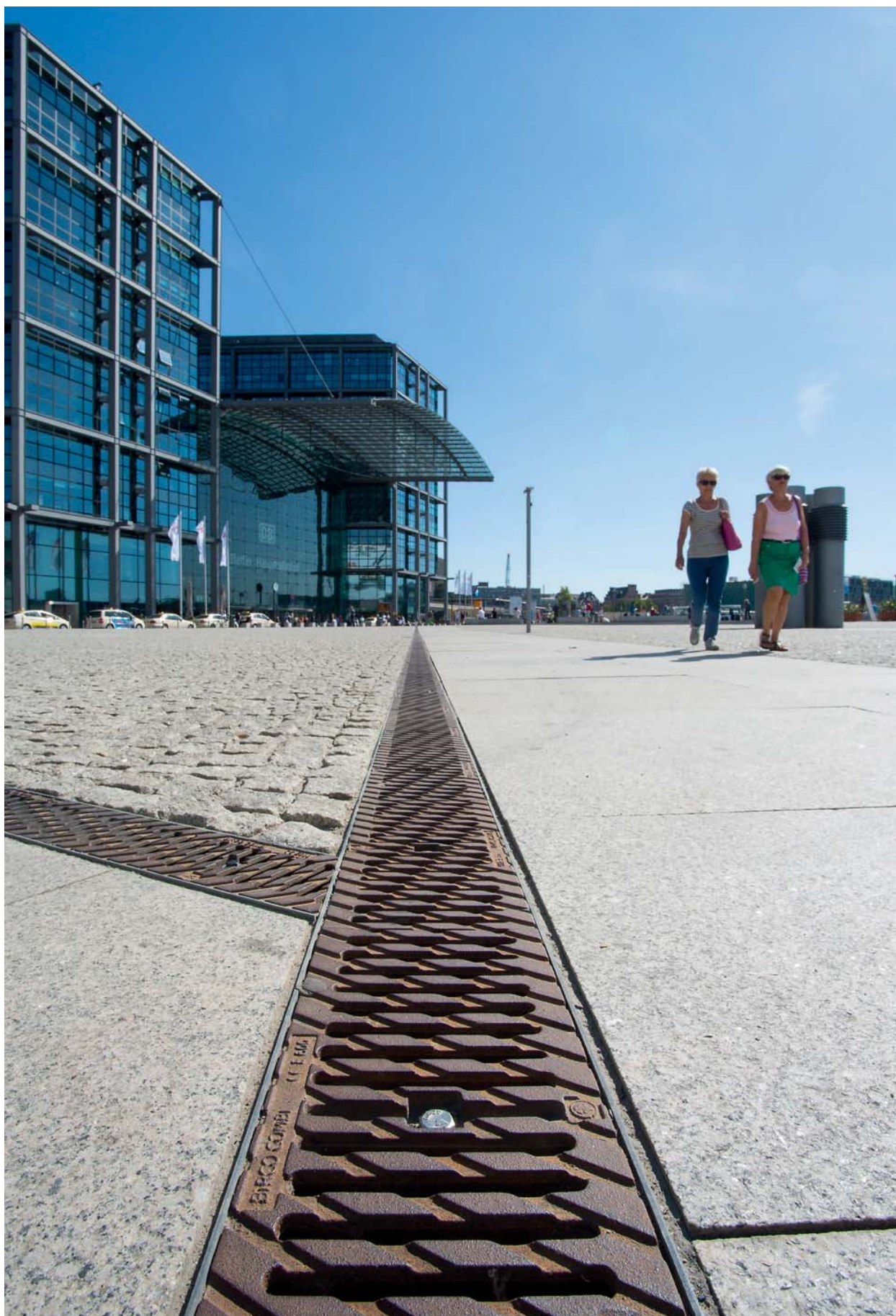
BIRCOLight op Washingtonplatz in Berlin
